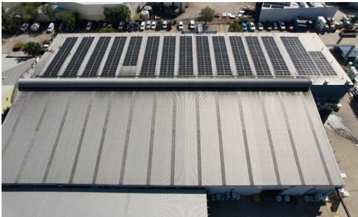
Solar panel installation at the Darra plant in Australia
