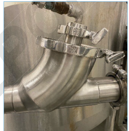
Figure 3. Ball Check Valve 1
