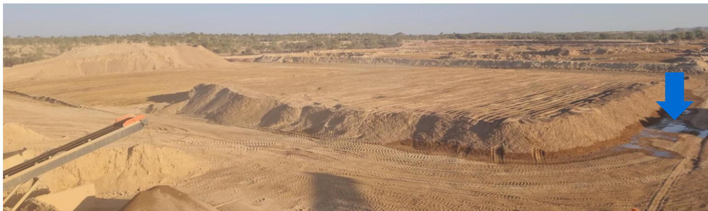
Figure 3 – Nalco Water FilterMax 88251 is still working in the final drying area, as evidenced by the presence of filtrate release. The pressure at the bottom of the stockpile is forcing more water to flow out
