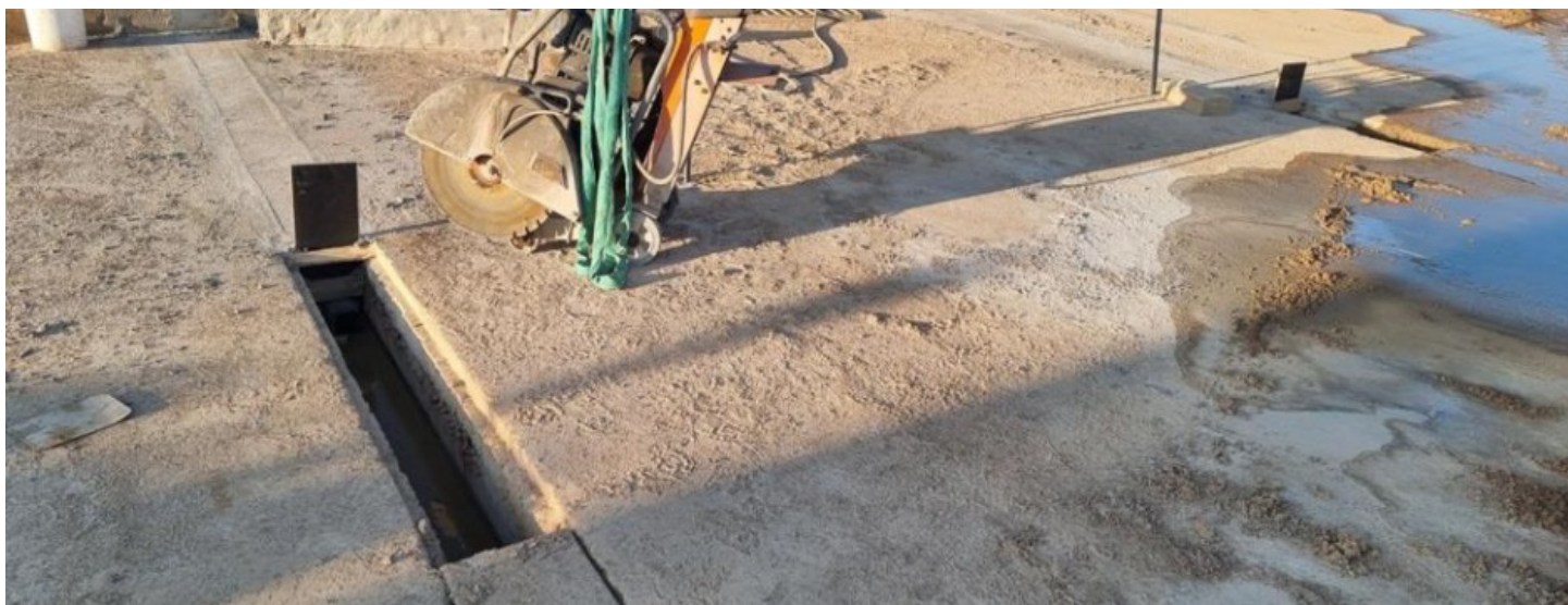
Figure 4 – Here the concrete pad drainage grates are being cleared to remove the free-draining water from the stockpile to keep the moisture down
