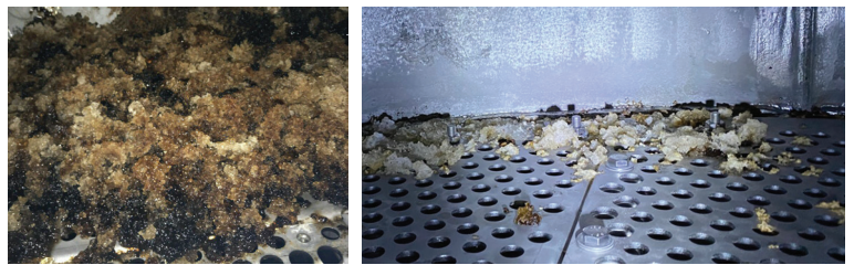
PHOTO 1: Column inspection during turnaround - Blank (left) and ACRYL-EX (right)
