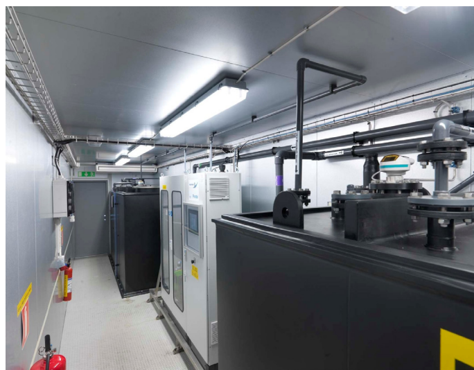
Fig.3 - Inside view of PURATE container showing control panel and chemical storage tanks
